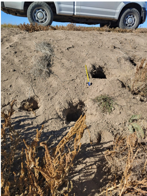
Photo of canal with weeds and animal burrows in KID.
