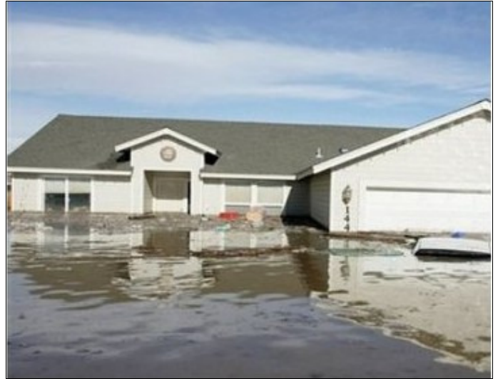
A newer Prairie Street home was among the hardest-hit properties during the January 5 flood in Fernley.
